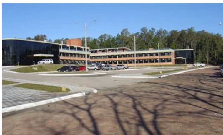
SOUTHERN REGIONAL SPACE RESEARCH CENTER – CRS/INPE Panoramic view of the main building of the at Santa Maria, RS, Brazil
